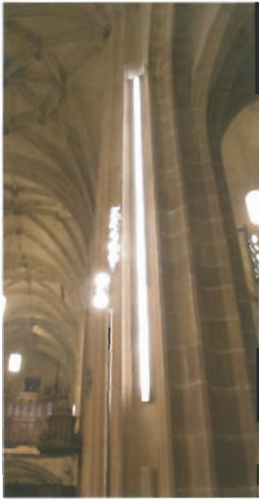
Viewing the altar from the pews, the observer is not affected by glare from the luminaires mounted on the columns. This is not the case for the priest, choir and servers.
